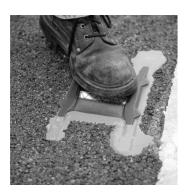
Adhesive may flow u and onto the front lip of the marker. If excess adhesive flows up in front of the reflective lens of the marker, remove he adhesive using a moist cloth, using care to prevent any of the adhesive from contacting the reflective lens. Adhesive on the lens of the marker will reduce reflectivity performance.
